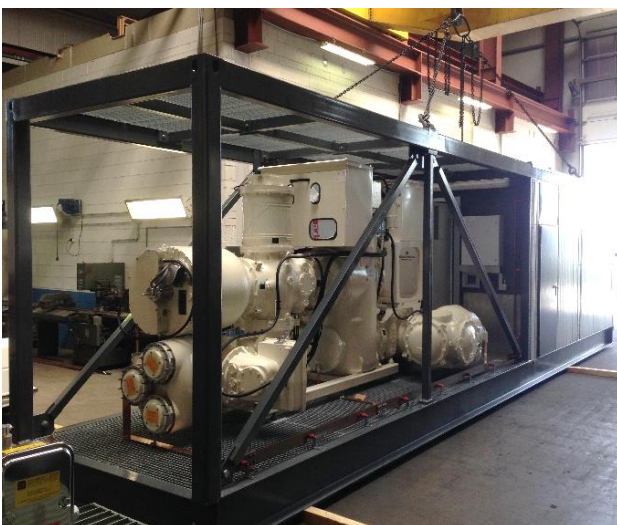
Fig. 4. Current construction status of the grid impedance measurement container
