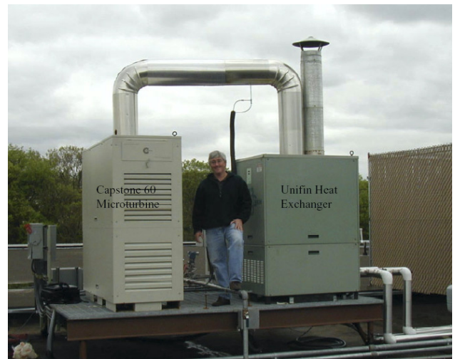
Figure 1. Capstone C60 microturbine with unifin heat exchanger
