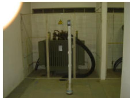
Fig. 1. Transformer cell and measuring instrument
